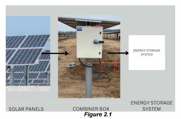
Figure 2.1 – Illustrated Example Usage of the Photovoltaic Combiner in an Energy Storage System Application
